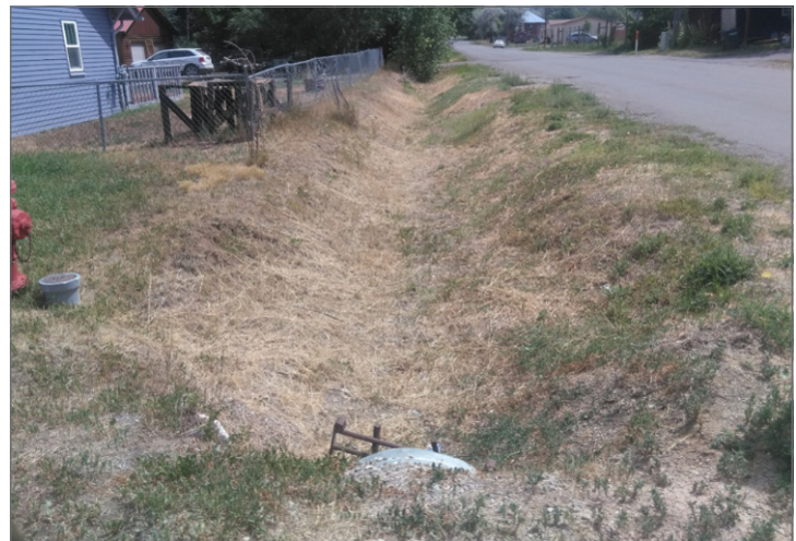
Figure 7-1: Typical Culvert and Ditch System Along South Spruce Street
