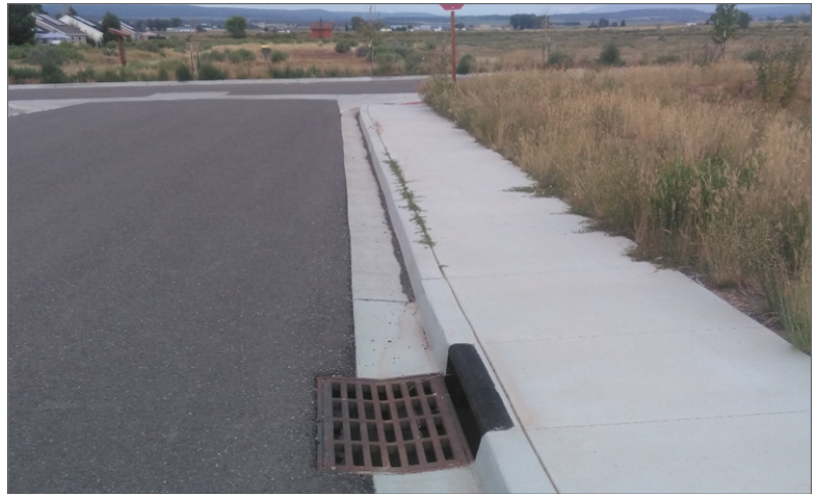
Figure 4-2: On-Grade Combination Inlet on Kiwi Street
