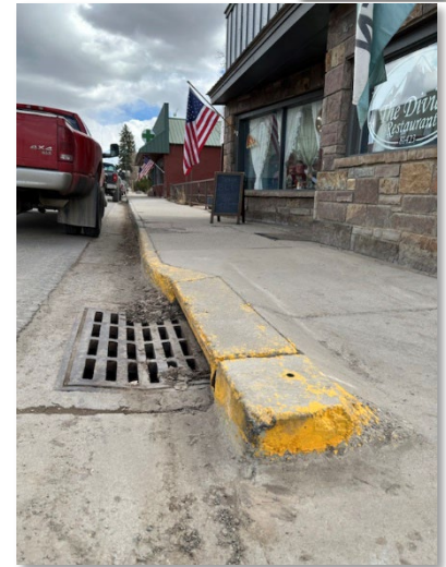
Storm drain inlet at Grand Avenue and Lucerne Street.
